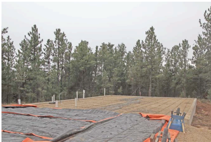
Black Hills Foundation Prior to Pouring Floor
