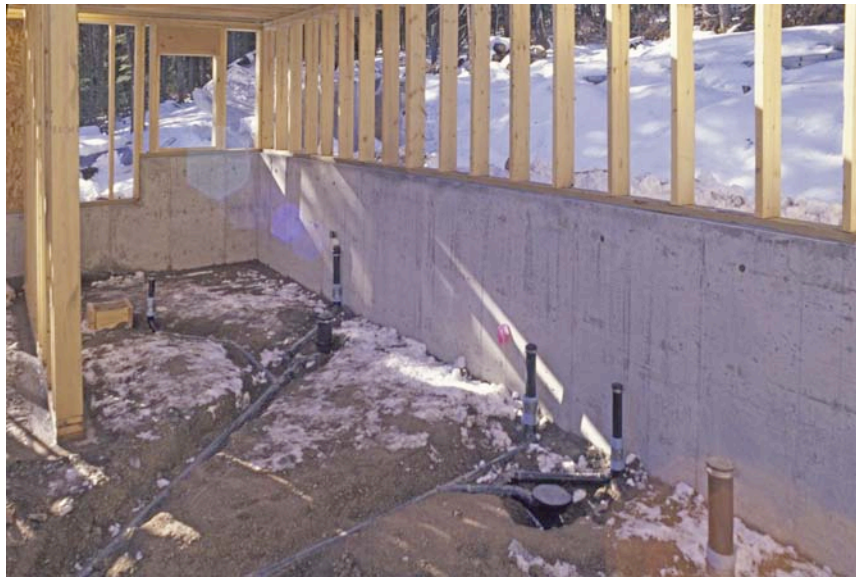
Underground Plumbing Ready for Inspection for the Bathroom and Laundry Area. Day Plumbing from Indian Hills did great plumbing work in the Denver foothills.
