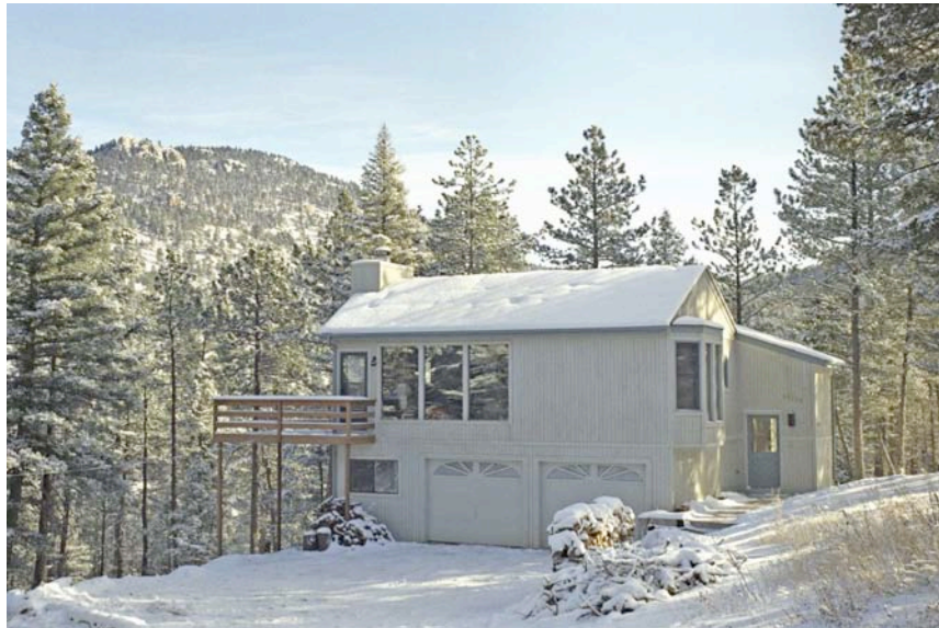
T1-11 Painted Siding on an Evergreen Home
