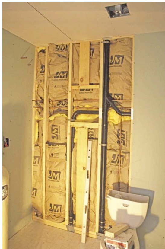
Bathroom Installation for the “Garage” Home
