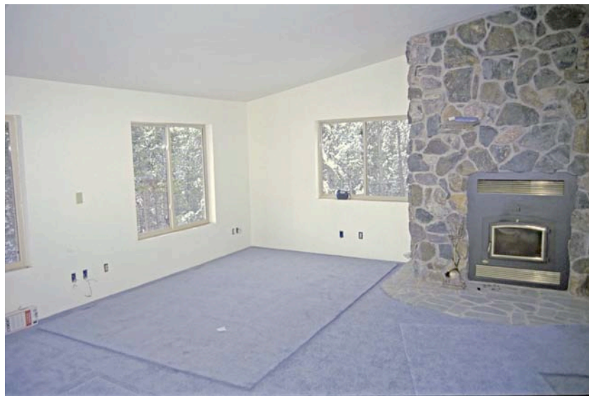
Carpet in the Process of Installation after Painting and Floor Tile is Completed
