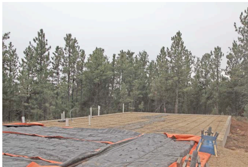
Black Hills Foundation Prior to Pouring Floor
