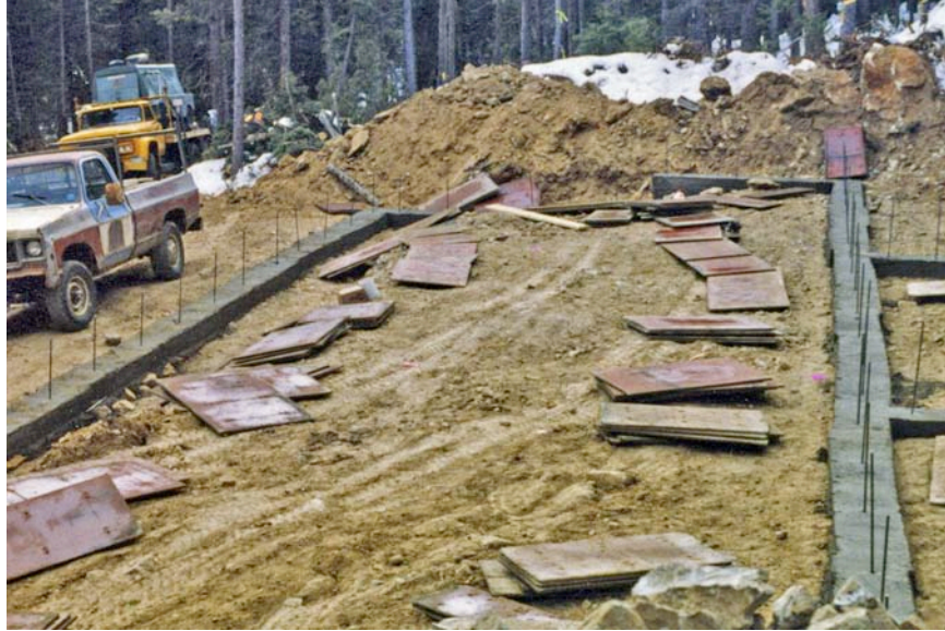
Footers for the Foundation Wall.
