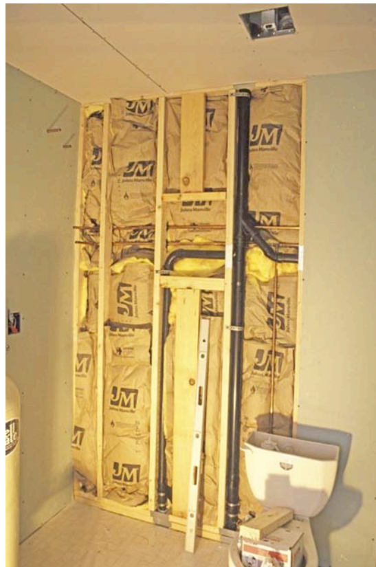
Bathroom Installation for the “Garage” Home
