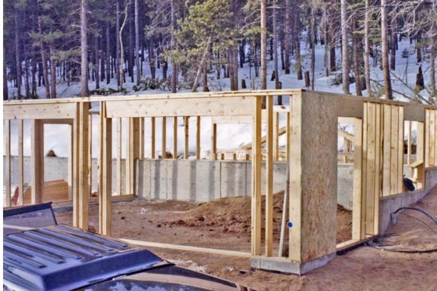
Start of Framing for a “Garage” Home.
