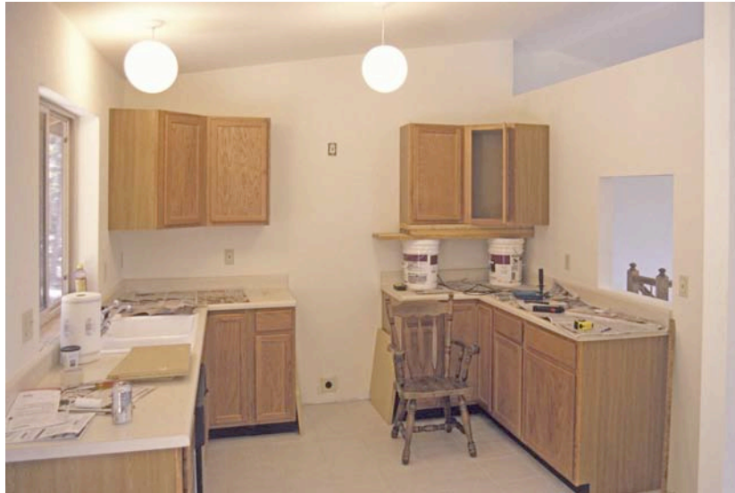
Kitchen Cabinets can be Installed after the Floor Tile is in Place and Walls Painted.
