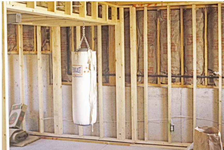
A Steel I-beam (just above the punching bag that is difficult to see) at my 1 st Home.
