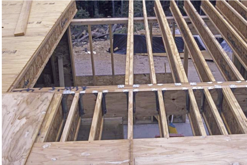
TJI Floor Trusses Installed
