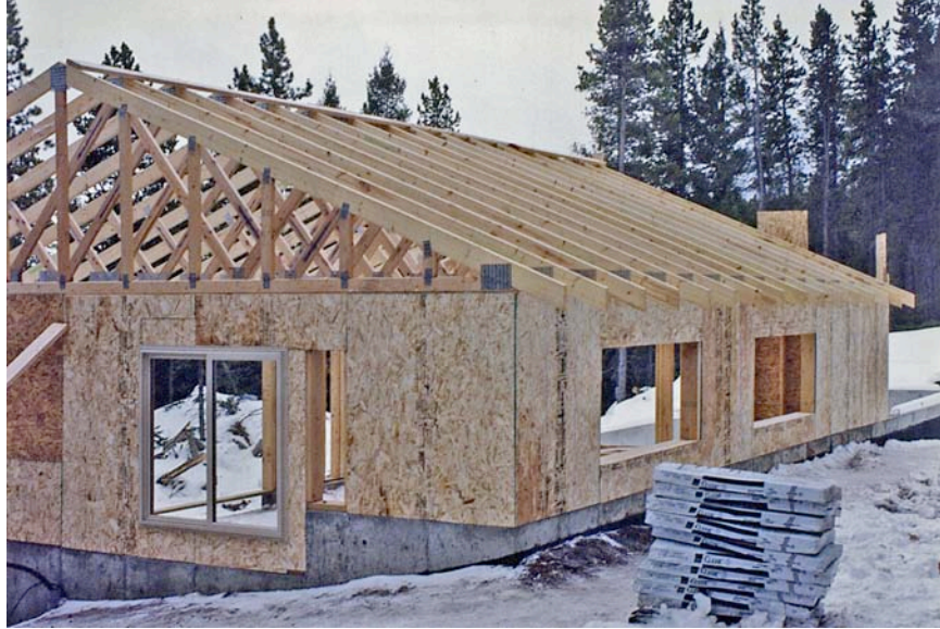
Pre-built Roof Trusses.
