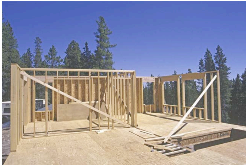
Start of 2 nd Floor Walls
