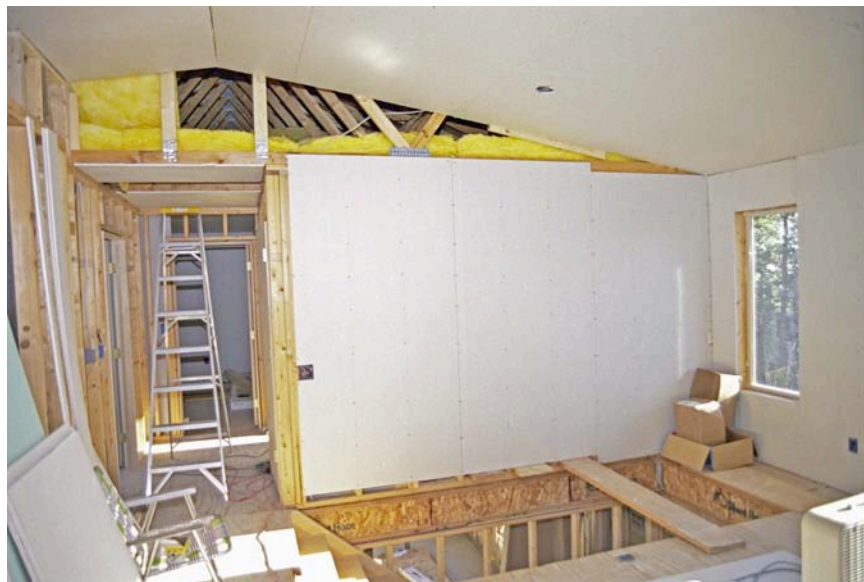
Drywall Installation
