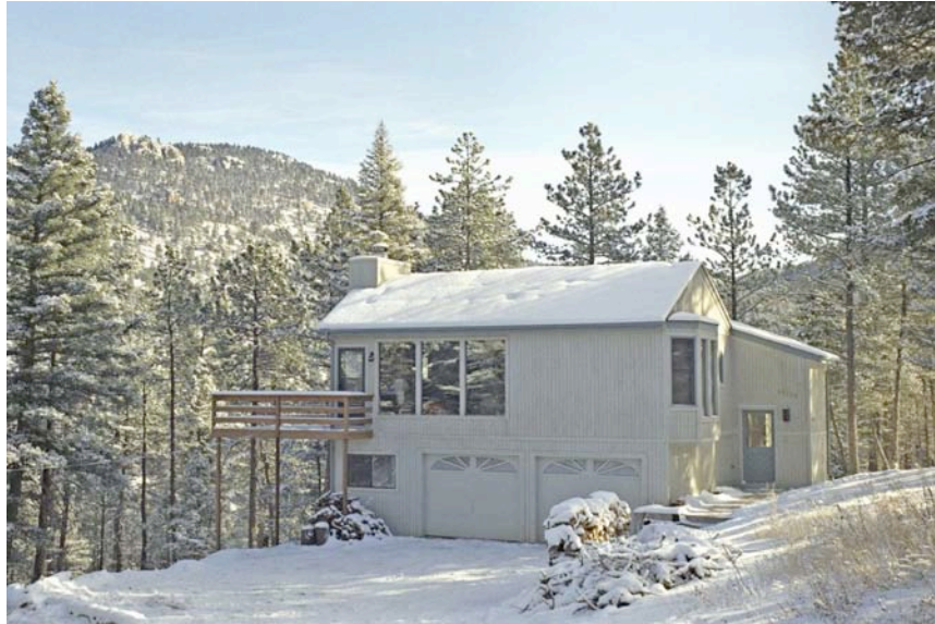
T1-11 Painted Siding on an Evergreen Home
