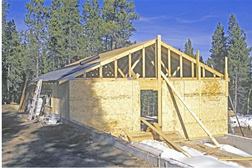
Start of Roofing for a “Garage” Home
