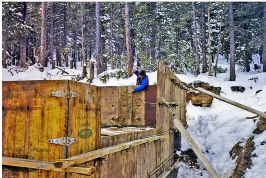
Footers for the Foundation Wall.
